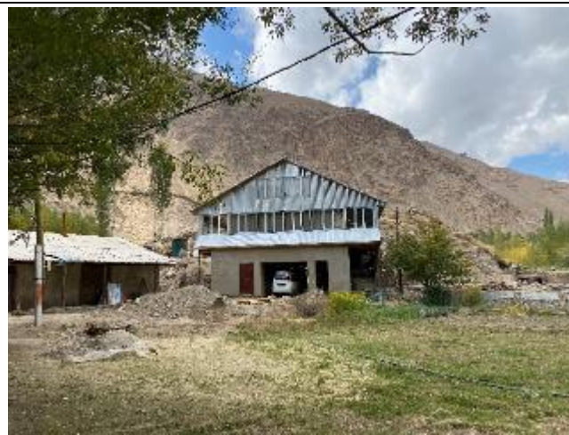
Photo 110: Newly built houses for resettlers near the intake
