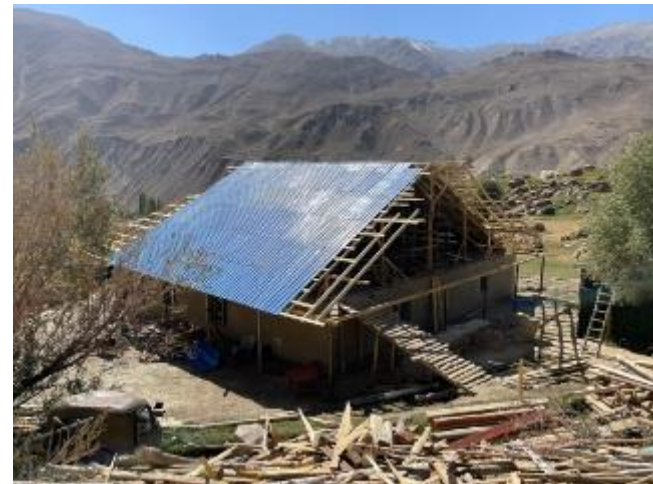
Photo 118: Nearly completed home at Upper Chagev
