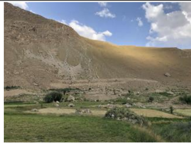
Photo 73: Terraces to protect Upper Chagev from rockfall
