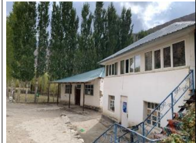
Photo 108: Business buildings in Barjingal village that will be relocated
