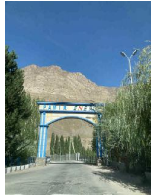
Photo 15: Gate to PEC main office and Khorog HPP
