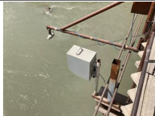
Photo 28: Flow gauge at old bridge
