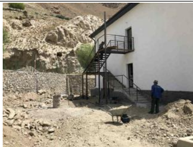
Photo 47: Finishing works at PEC Sebzor building
