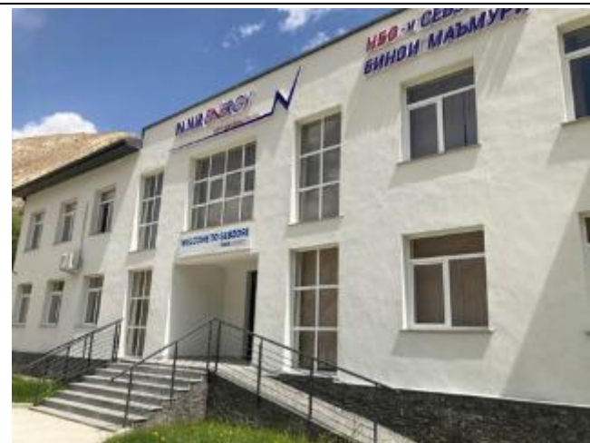
Photo 46: PEC Sebzor administrative building
