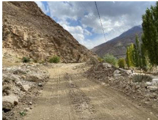
Photo 119: Temporary spoil and material storage area
