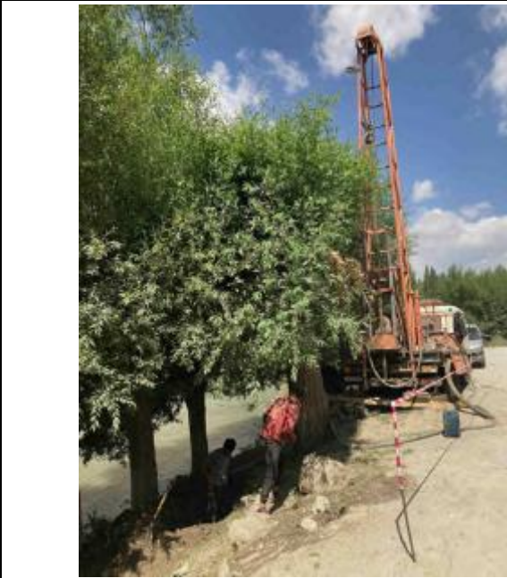
Photo 32: Test drilling at bridge upstream of intake
