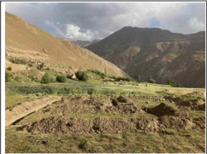
Photo 69: New home site preparation in Upper Chagev
