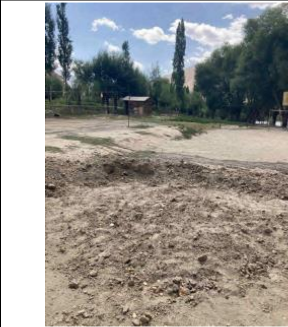
Photo 31: Refilled test pit at school
