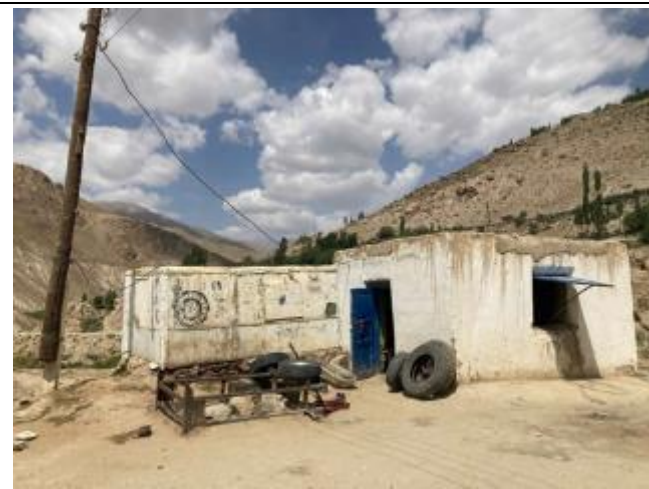
Photo 37: Roadside tire business at intake
