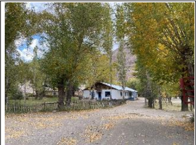
Photo 111: One of the old school buildings located above the reservoir and to be rebuilt at higher elevation
