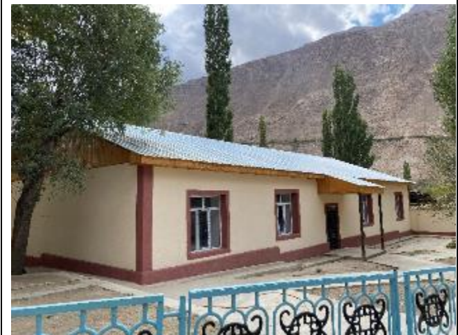
Photo 114: Refurbished education and cultural centre, to serve as temporary school
