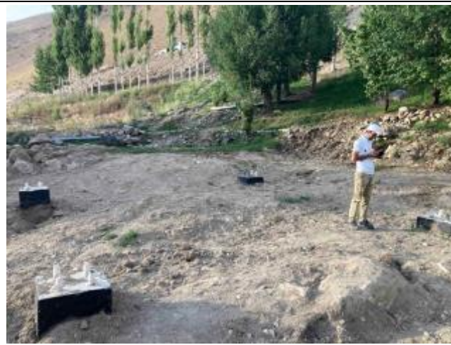
Photo 74: Transmission line tower foundations in Upper Chagev
