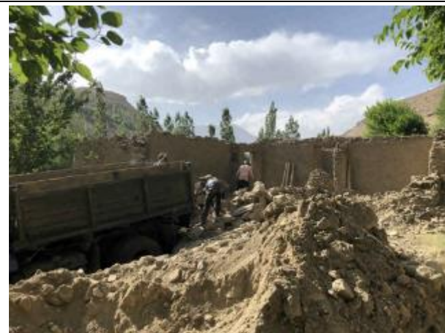
Photo 58: Demolishing of resettled family home at powerhouse
