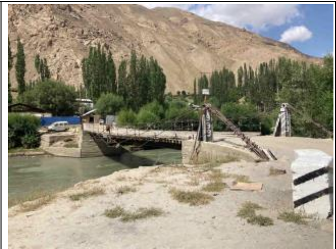
Photo 27: Old bridge upstream of intake
