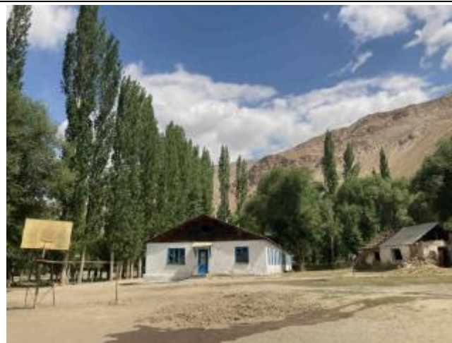
Photo 29: Old school on riverbank at reservoir
